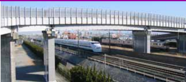
Arai Route12/Arai Overpass (Arai town)
