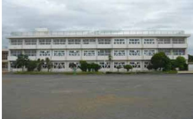
Fujiminami Junior High School Building (Fuji City)
